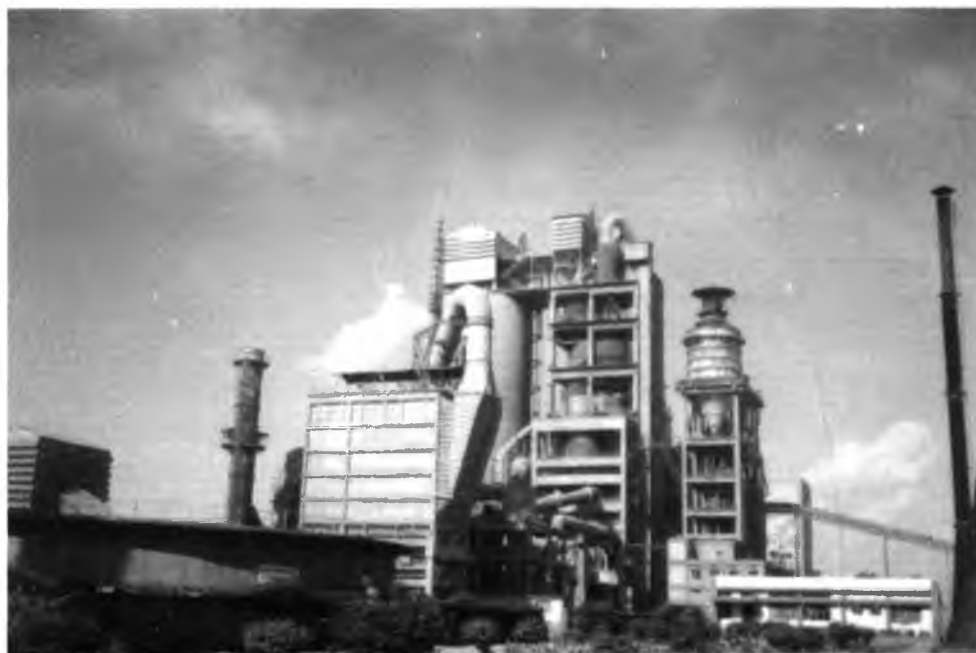
Modern Cement Plant
