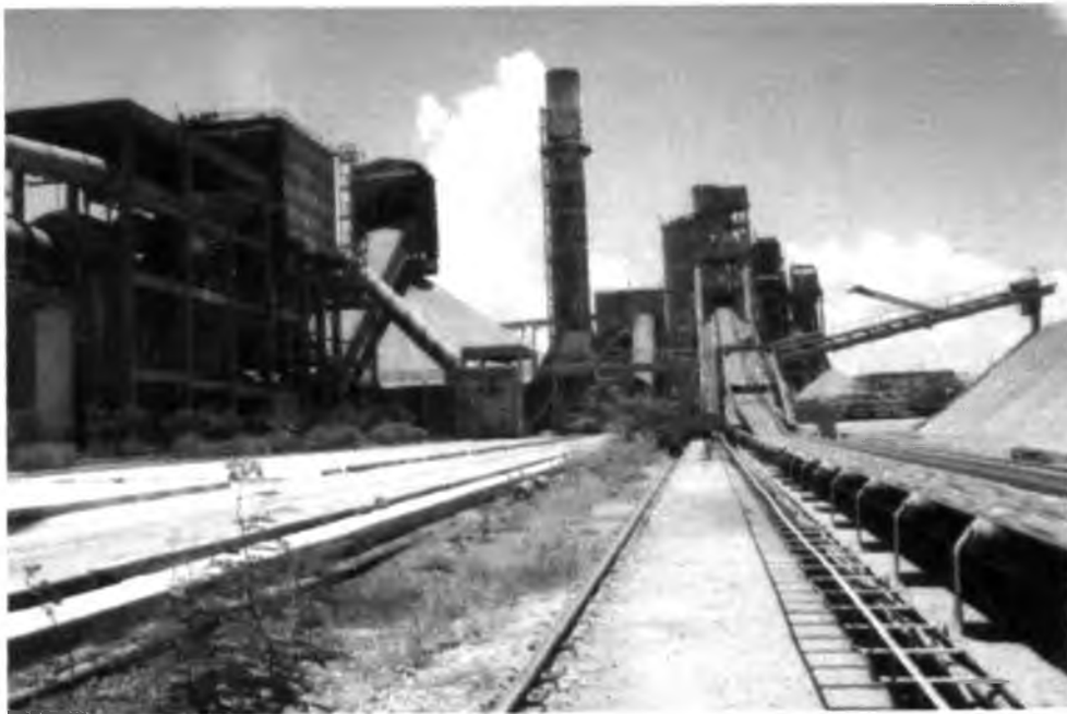
Limestone Stacker Reclaimer, Cooler, ESP & Chimney
