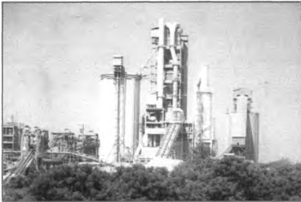
Environment-Friendly Modern Cement Plant
