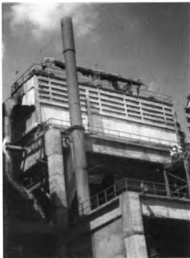
Bag Filter for Coal Mill
