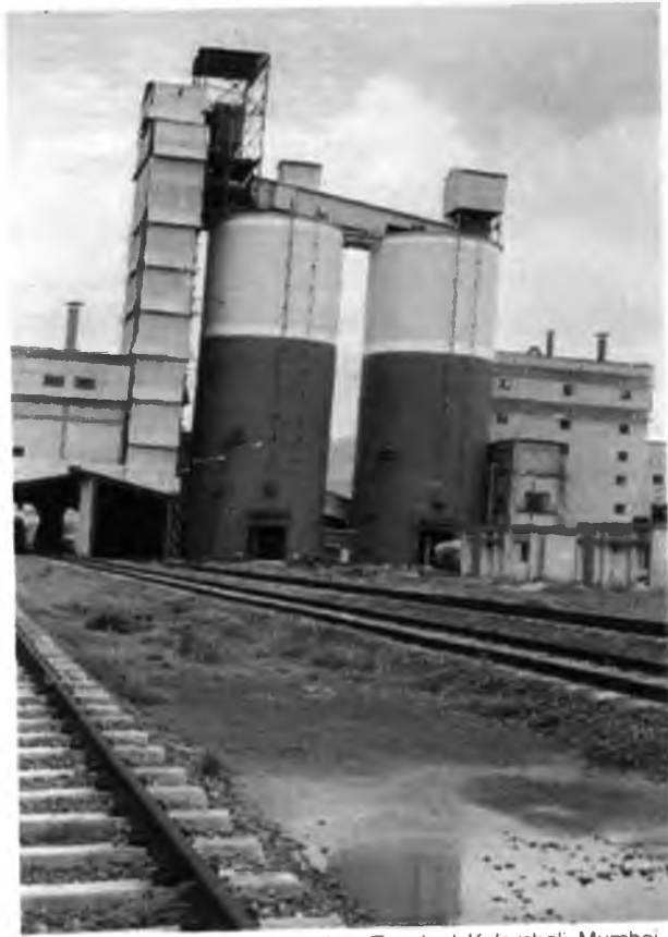
Bulk Handling Terminal, Kalamboli, Mumbai
